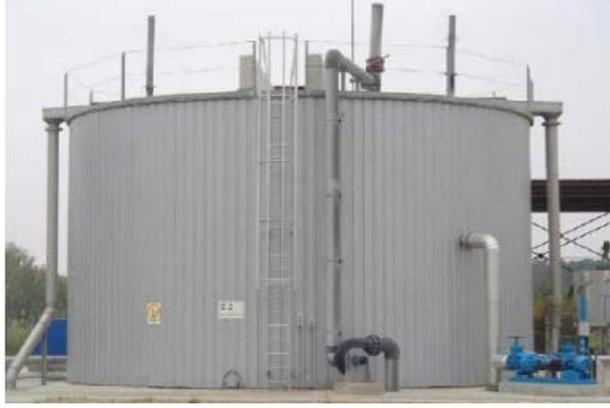
**Figura A5. Digestor ATAD**
