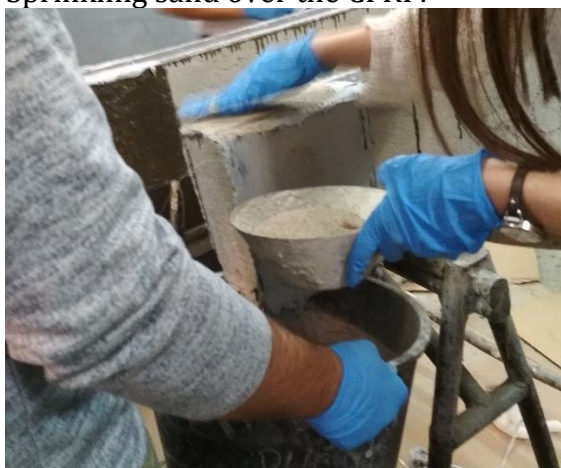
Sprinkling sand over the CFRP.
