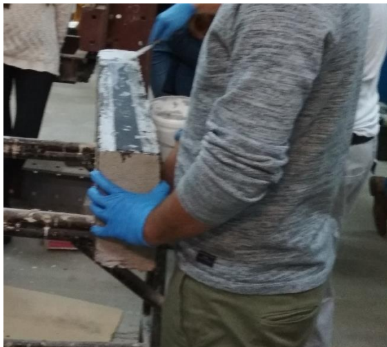
Cover the CFRP with more adhesive
