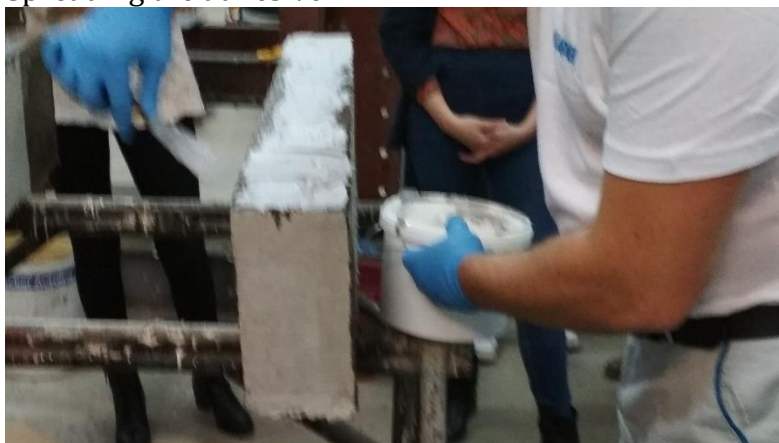
Spreading the adhesive.
